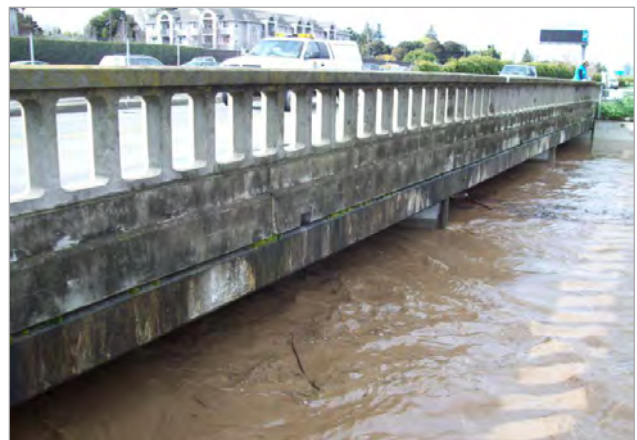
Flooding along San Francisquito Creek.
